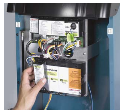
Installing an IQ Option Card
